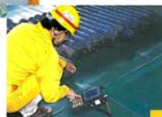
Ultrasonic testing of high temperature bolt
