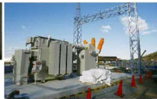
Installation work of facilities to receive extra-high voltage power
