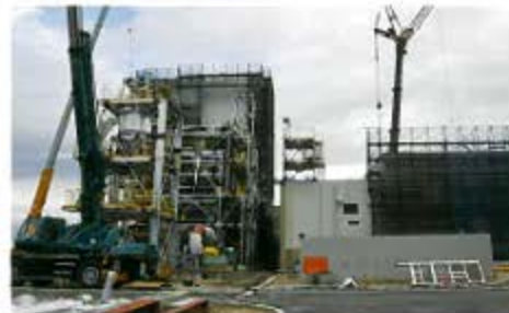
Construction work at our woody biomass power plant "Taki Biopower"
