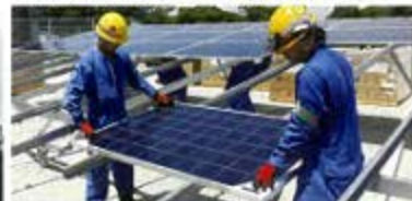
Construction work at photovoltaic power plant
