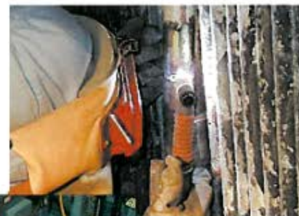
Evaporation pipe welding work
