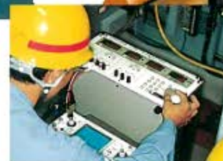
Test control of electrical equipment
