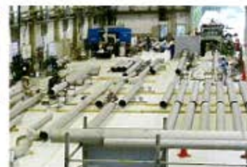
Status of pipe processing and finishing at Oe Plant No. 1
