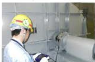
Rotary machine diagnosis in condition monitoring and maintenance work at Hamaoka Nuclear Power Station
