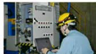
Control device installation work
